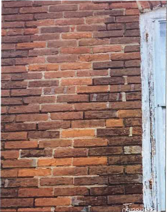
Areas of severe mortar deterioration.
