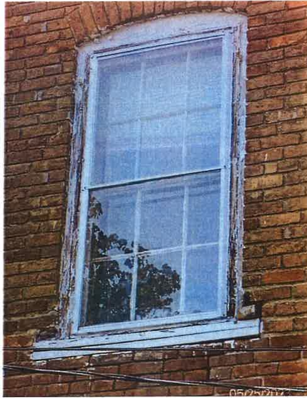
Additional examples of wood deterioration and loose bricks around windows.
