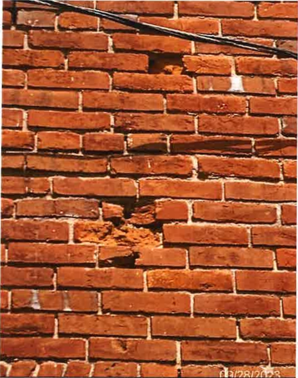
Areas of spalling brick.
