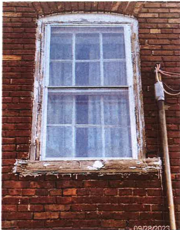
Additional examples of wood deterioration and loose bricks around windows.
